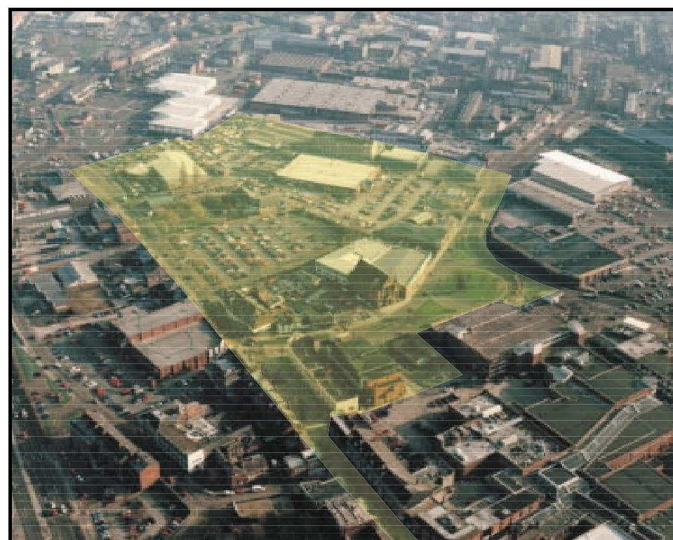
The Rock Triangle Development Area viewed from the west
